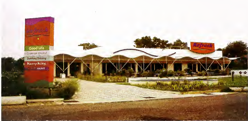
Fig. 21 View of a Roadside Rest Area along a National Highway
