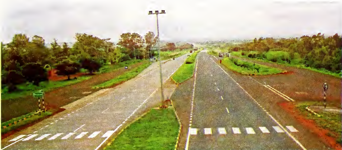
Fig. 24 Screen Plantation along Urban Highway
