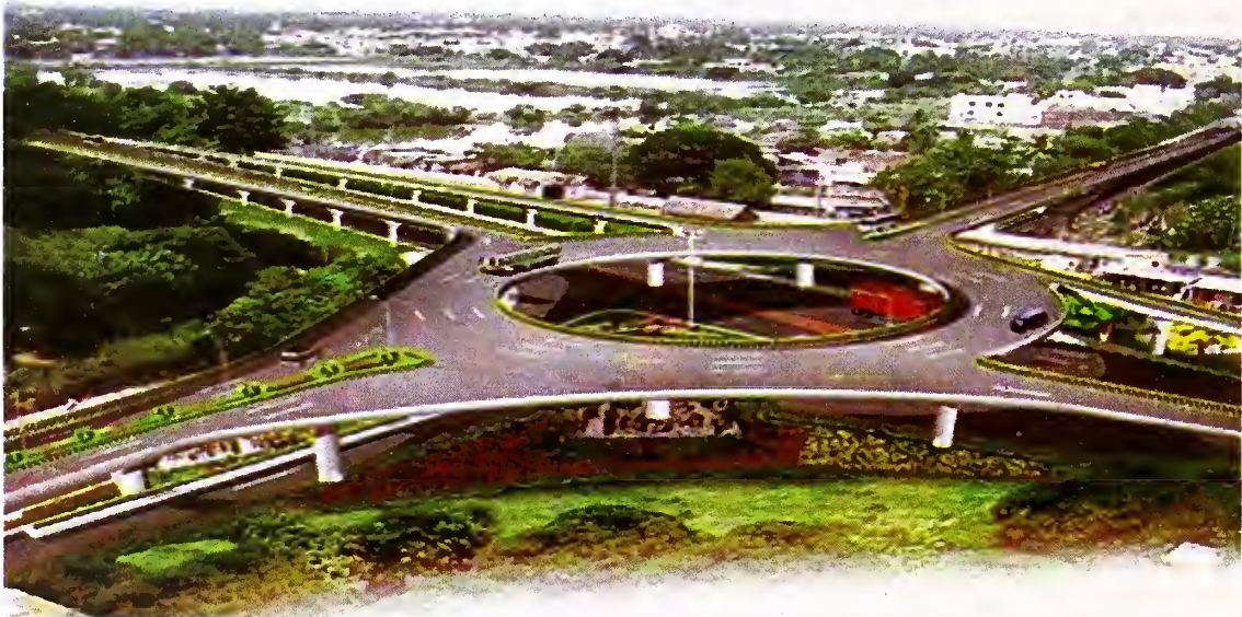
Fig. 18 Landscape Treatment of a Large Rotary and included Corners through various Measures
